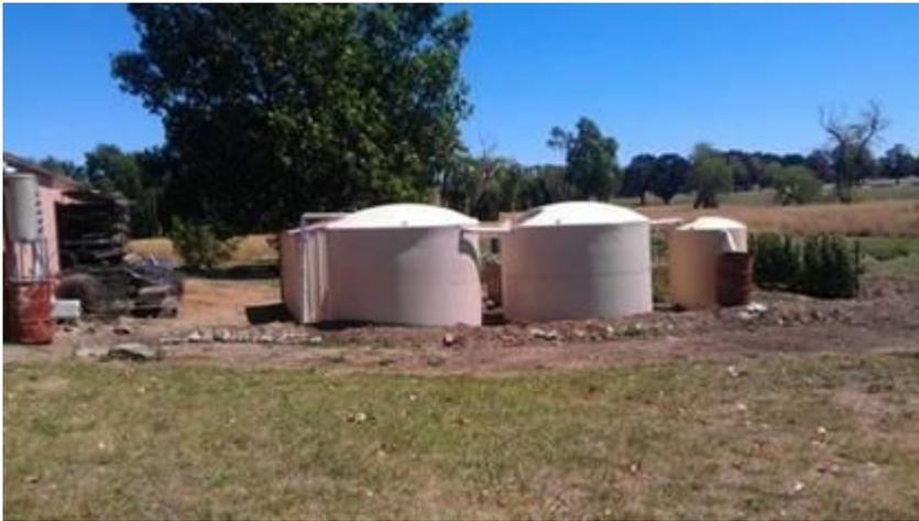
This ↑ is how the installed tanks now look with all the earthworks essentially complete. You will note that all the rubble (shale and rocks) and clay has been tidied up and the area will now be easily mown once the grass comes back. The earth mound will deflect excess water in a downpour that has, up until now, run through the garden and caused damage to crops and the garden layout. This photo was taken on Tuesday 15/1.
